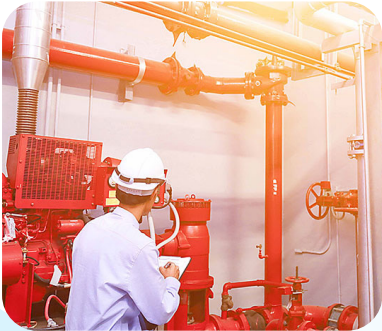
Fire Safety Works
