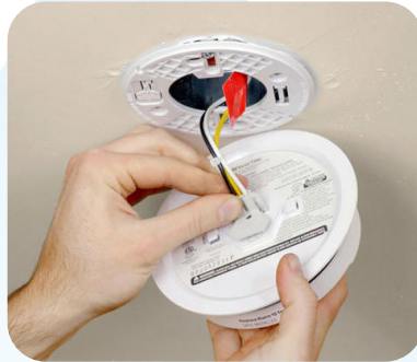
Fire Alarm & Smoke Detector Installation
